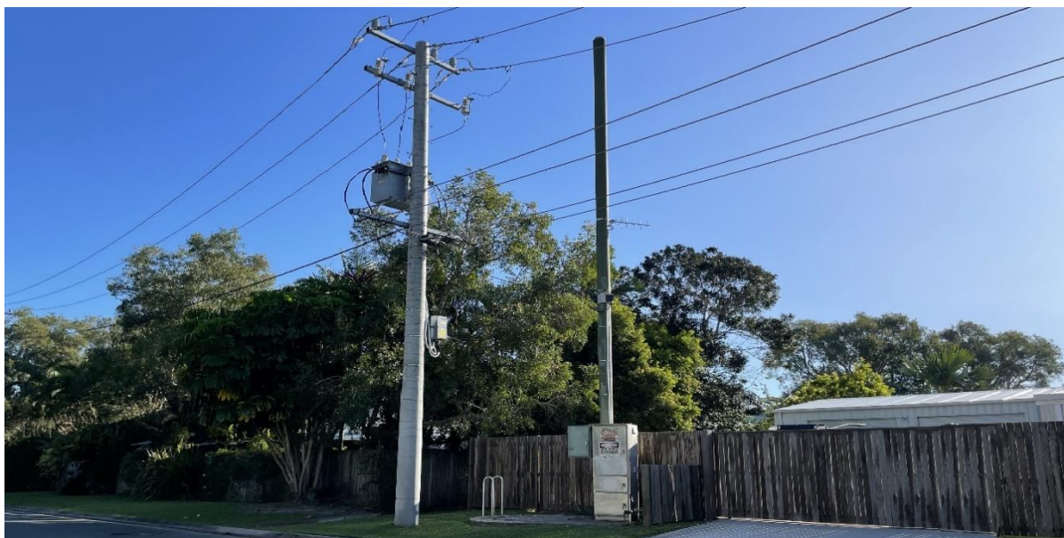
Figure 12. The pumps in this well can only be safely lifted after Energex has attended and isolated the overhead lines.
